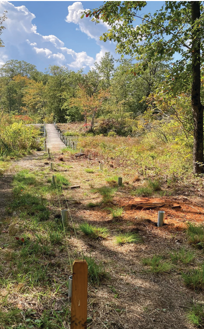
Boardwalk under reconstruction
